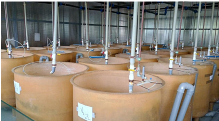
Fig. 2 - Recirculating aquaculture system (RAS) tanks with the experimental batch of fish
