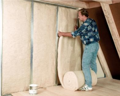
Photo 1. Wool mattresses for wall thermal isolation
