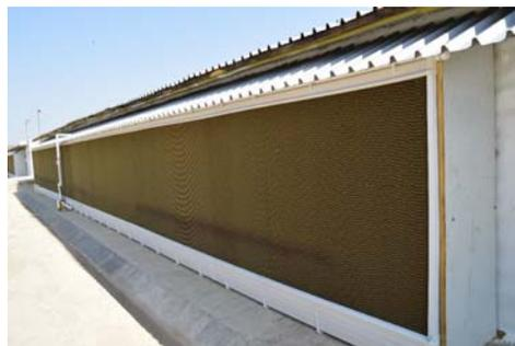
Fig. 4 Cooling pad cooling system used in the FermaDor unit (original photo)
