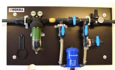
Fig. 3 Mechanism of water pressure regulation and dosing of substances in water in farmhouses 7-8 FermaDor
